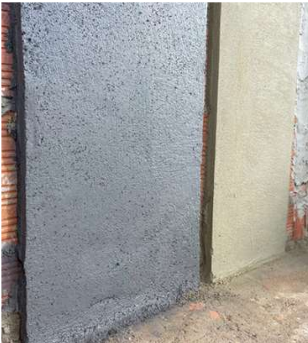
Figure 4. Application of 1 m 2 of BEM and other cement mortar.
